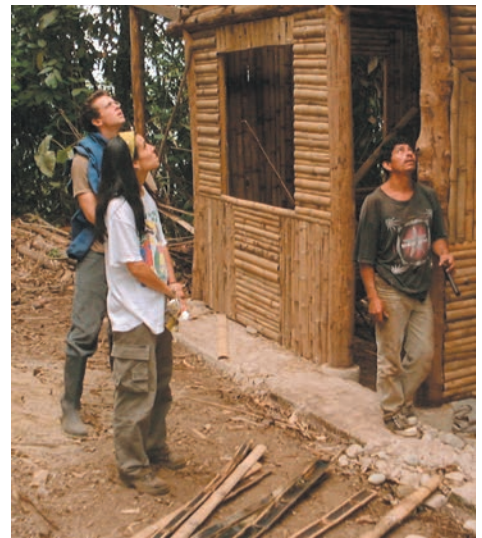
Progress on the new refuge at Junin
