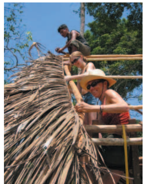
Volunteers help to repair a roof at Playa Larga
